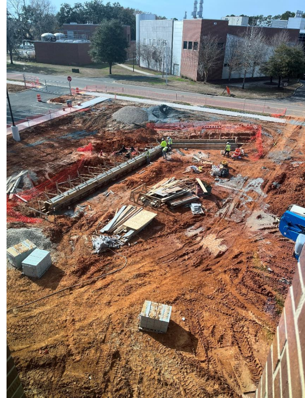
Site work looking west (impacted by sink hole discovery)
