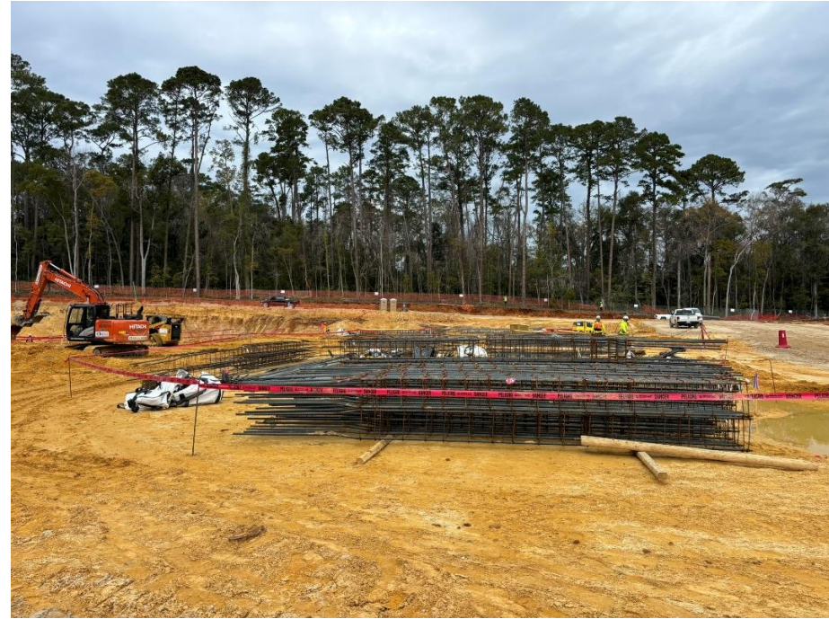
Pre-tying rebar for columns for faster installation
