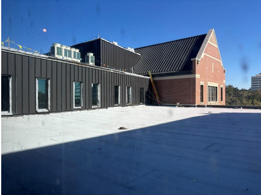
Roofing nearly complete all areas
