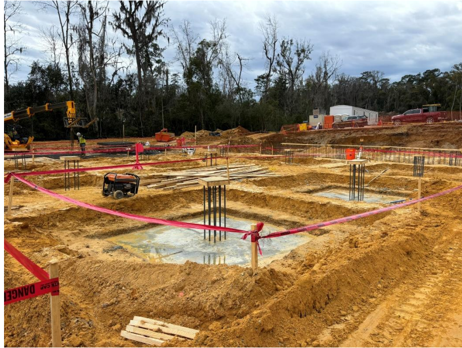
Concrete placement for foundations in process
