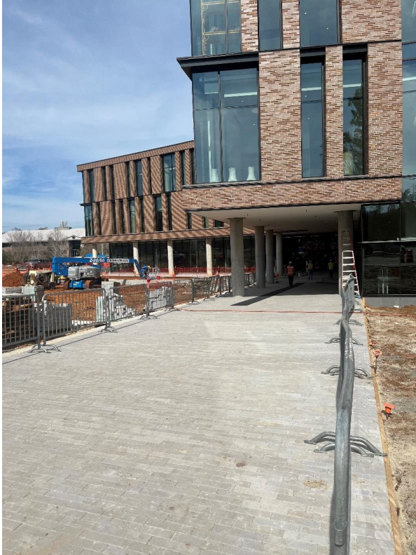
Brick paver installation 95% complete
