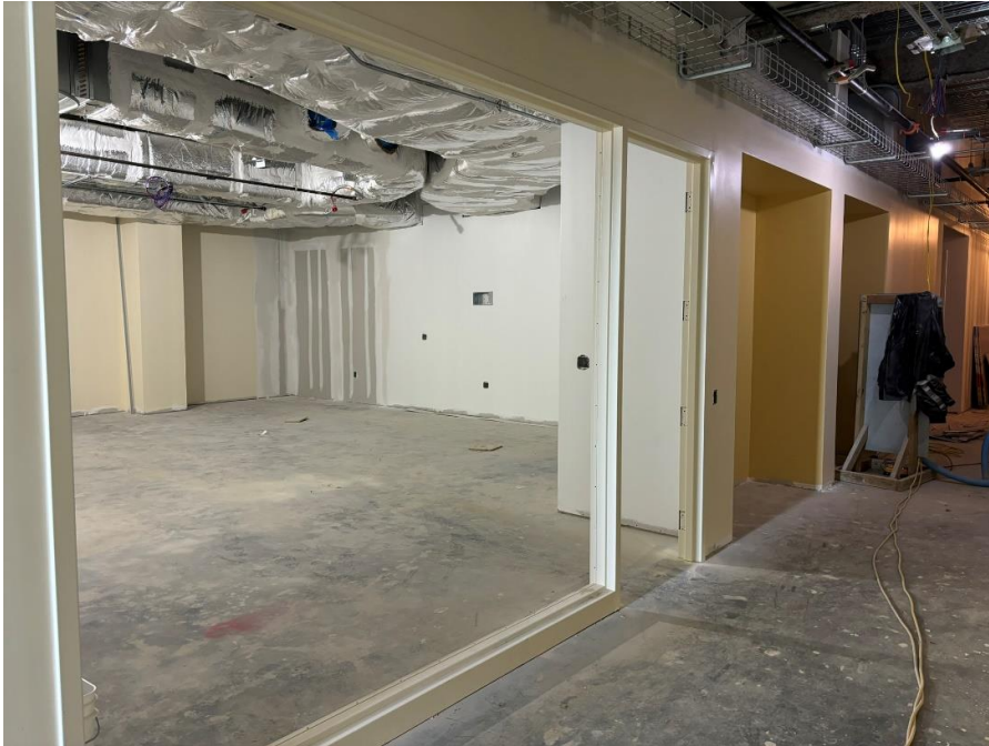
Office area – typical view
